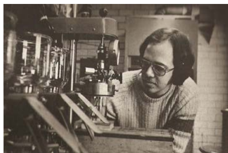
Mike Prudich investigates the removal of ash particles from liquefied coal by partitioning the particles into a water phase.
