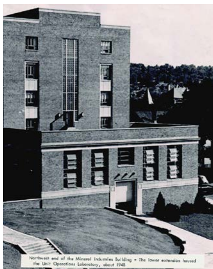
Northwest end of Mineral Industries Building – The lower extension housed the Unit Operations Laboratory – 1948
